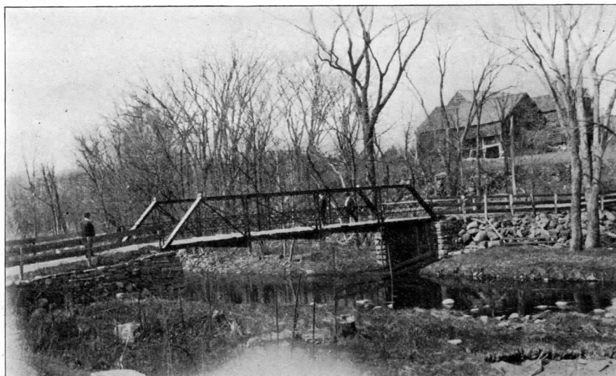
Alplaus Kill — \frac{1}{4} Mile above Dam Site. Buildings on right will be submerged by Proposed Reservoir.
