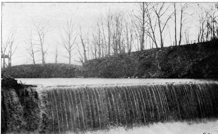
Alplaus Kill at High Mills Dam.
